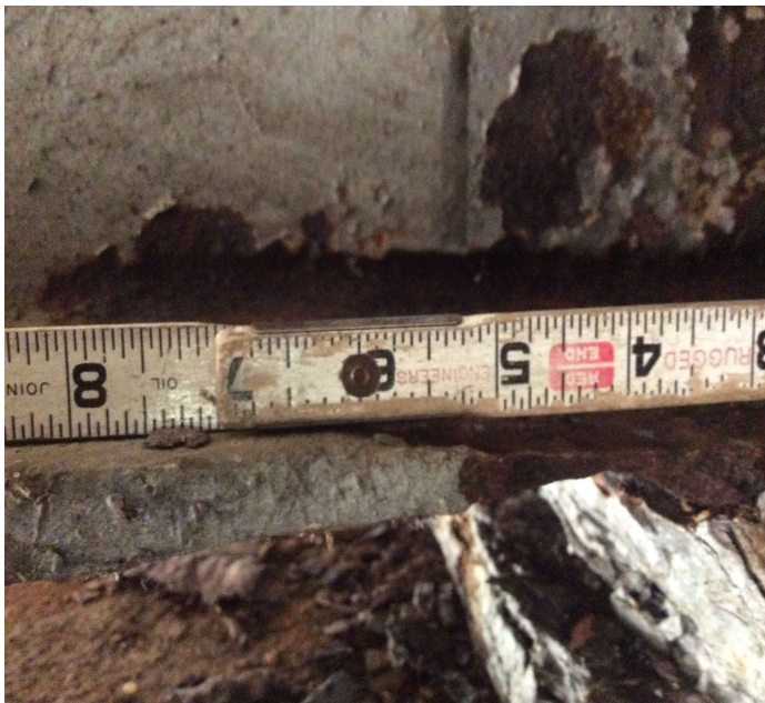
PHOTO 1 Description Bent 5 girder 4 section loss up to knife edge on bottom flange at bearing area right side girder.
