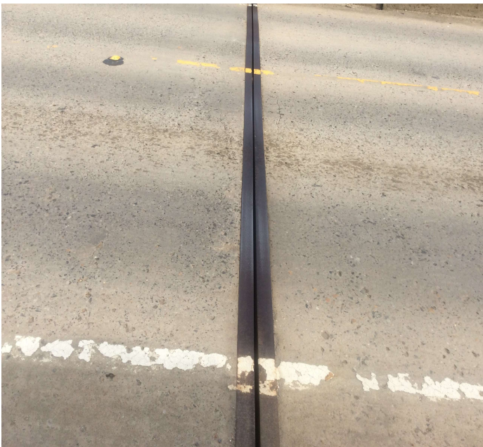
PHOTO 1 Description Joint seal at bent 3 is missing.
