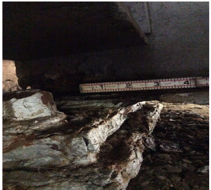
PHOTO 2 Description Bent 5 girder 4 section loss up to knife edge on bottom flange at bearing area left side of girder.
